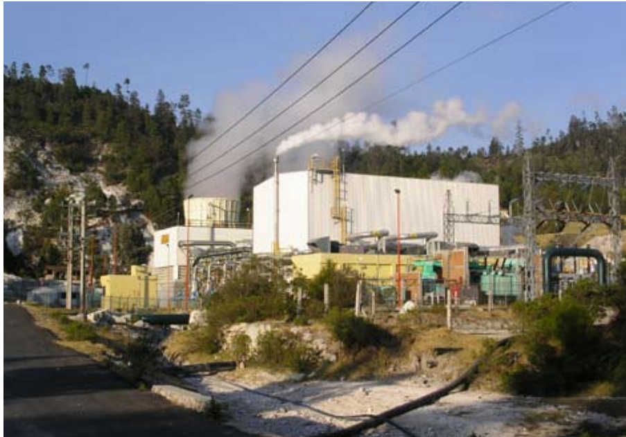
Illustration 10. Geothermal power plant in Los Azufres, Michoacan
