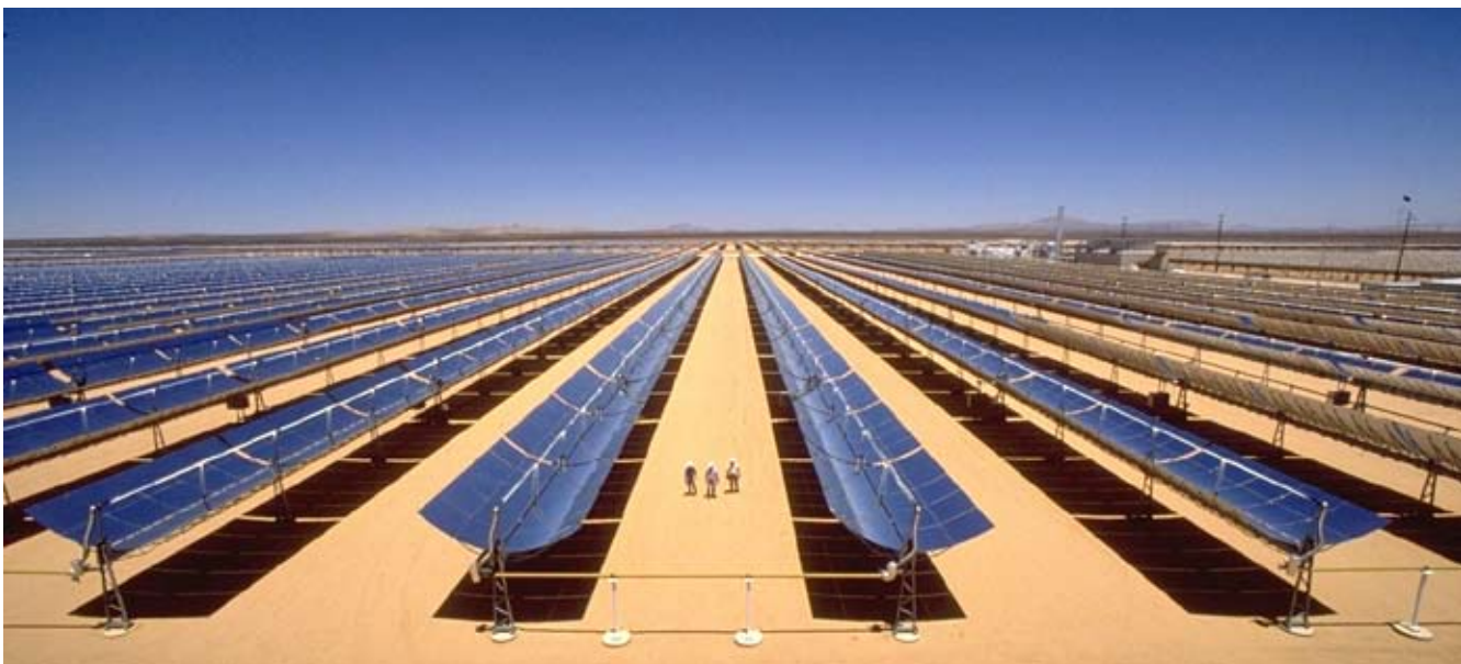
Illustration 5. Parabolic trough power plant Kramer Junction, California
