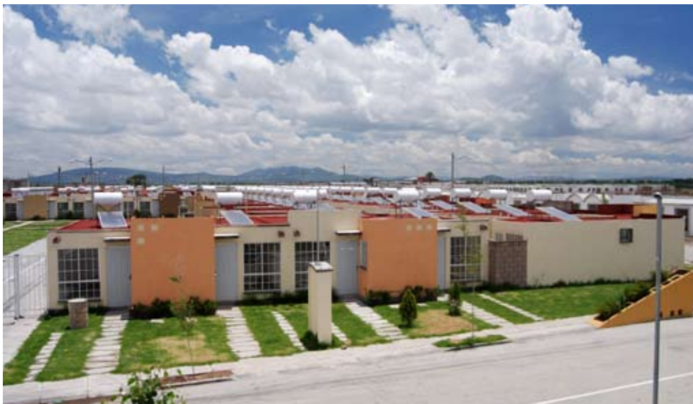
Ilustración 12. Solar water heaters in household applications
